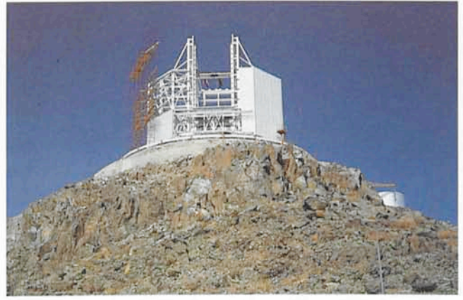
Figure 3: The rotating building under construction in April 1988.
