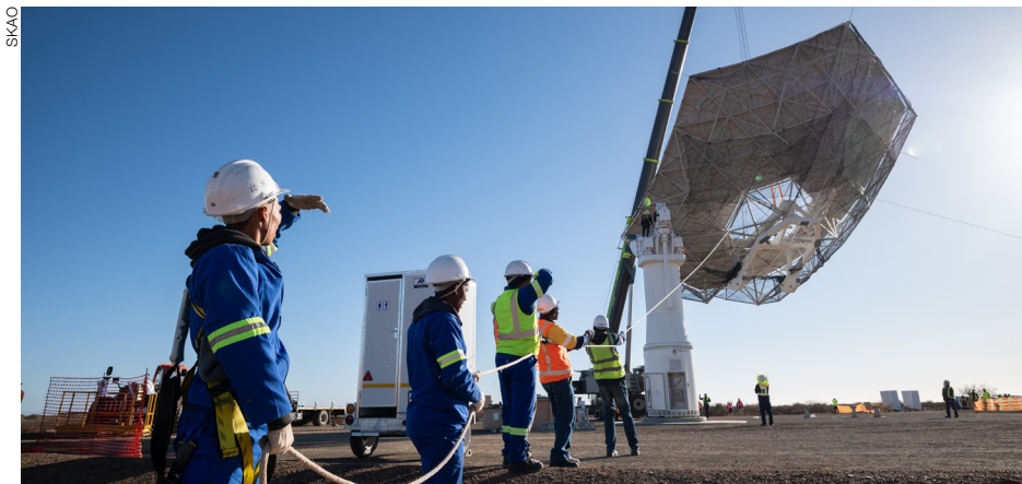
The 'big lift' of the main reflector onto the pedestal of the first SKA-Mid production dish on site in South Africa. The lift took place on 4 July 2024, and was carried out by a team from the SKAO, South African Radio Astronomy Observatory (SARAO) and China's CETC54.
