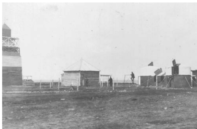
Figure 7: Photograph of the German station in Punta Arenas. Left, wooden lighthouse of Punta Arenas, center, "tea house" and meteorological station, right, two observing domes made from iron and canvas (Archiv, Berlin-Brandenburgische Akademie der Wissenschaften).
