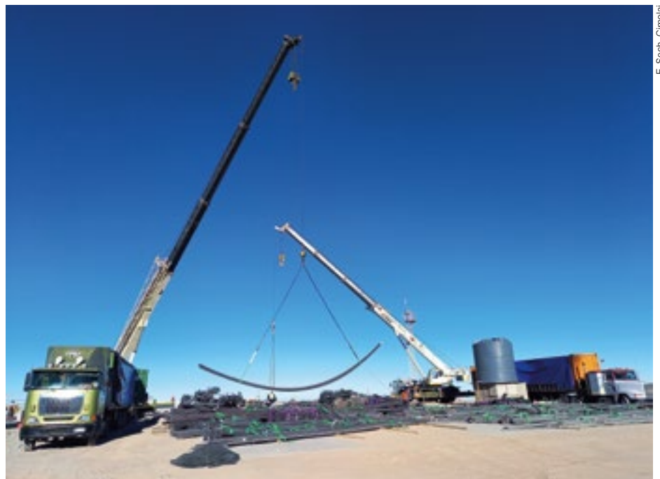
Handling of material and equipment received from Europe for the ELT Dome and Main Structure, Cerro Armazones.
