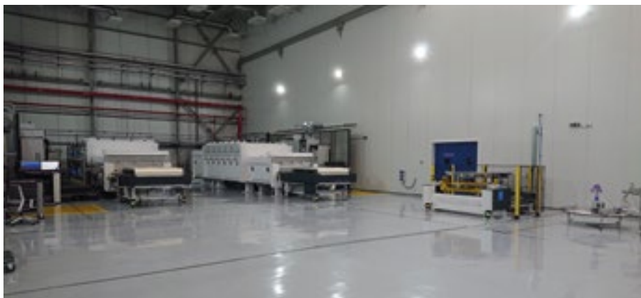
The installation of the first M1 segment coating plant started in February 2022 in the ETF at Paranal after more than a year and a half in storage because of the pandemic. By the end of the year, the two plants were operational. They will be used to coat the M1
