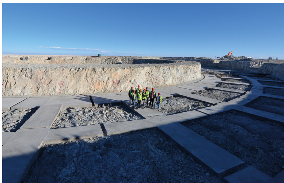
ESO staff members visiting the dome site upon completion of the excavation. Lean concrete has been poured on the rock and the opening to the 7-metre deep telescope main structure foundations can be seen behind the staff.
