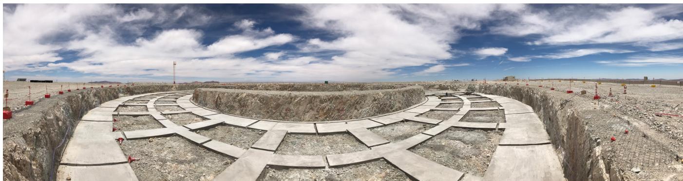
Panoramic view of the excavation for the auxiliary building which will surround the dome.
