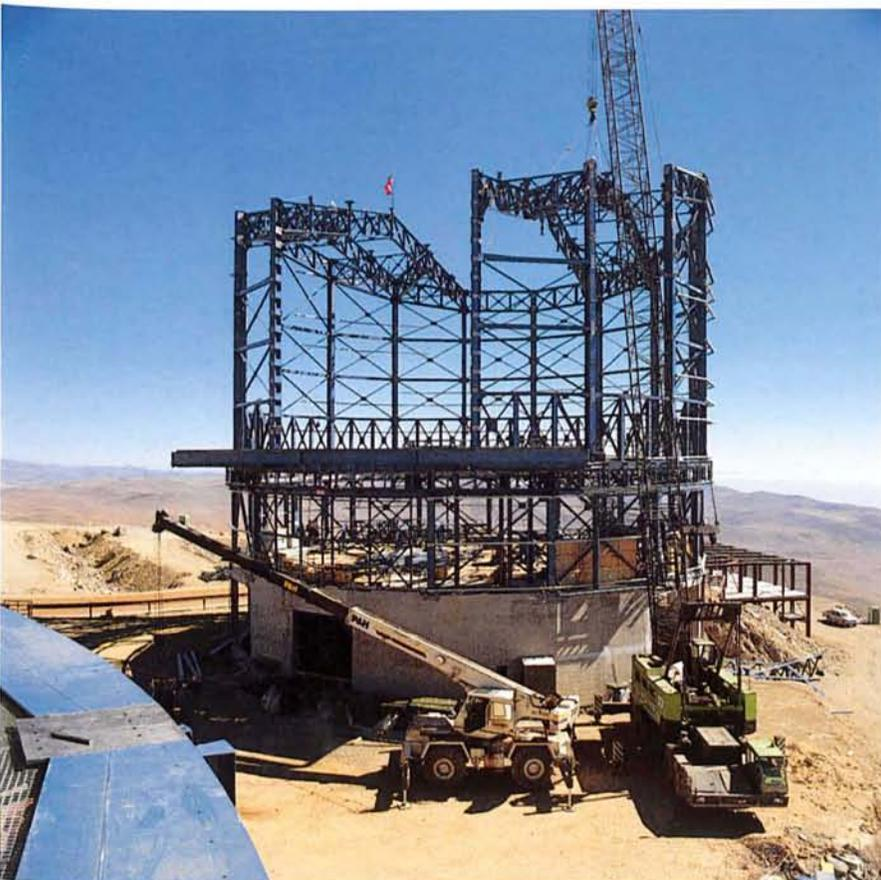
of the construction. The structure has a low-weight construction, specially designed to protect the telescopes from the strong desert wind.
