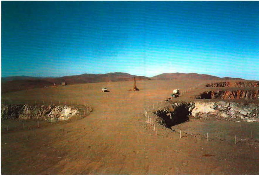
Figure 5: Overview of the Observatory site showing the telescope excavations and, in the centre of the "Platform" the equipment used to measure the GVTF. The view is taken from the north.
