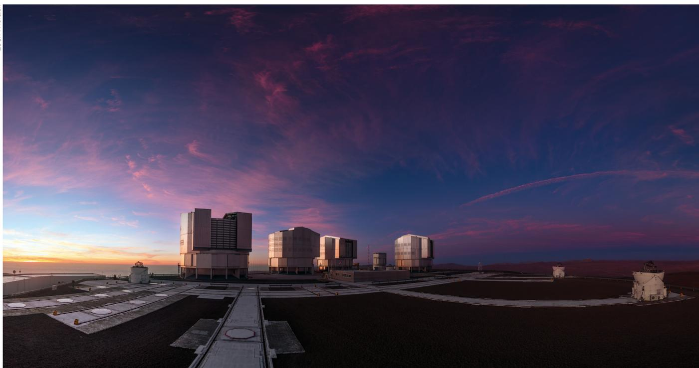
As the Sun sets, ESO's Very Large Telescope (VLT) springs into action to begin its nightly mission. Consisting of four 8.2-metre Unit Telescopes (UTs) — named Antu, Kueyen, Melipal, and Yepun — and four smaller 1.8-metre Auxiliary Telescopes (ATs), the
