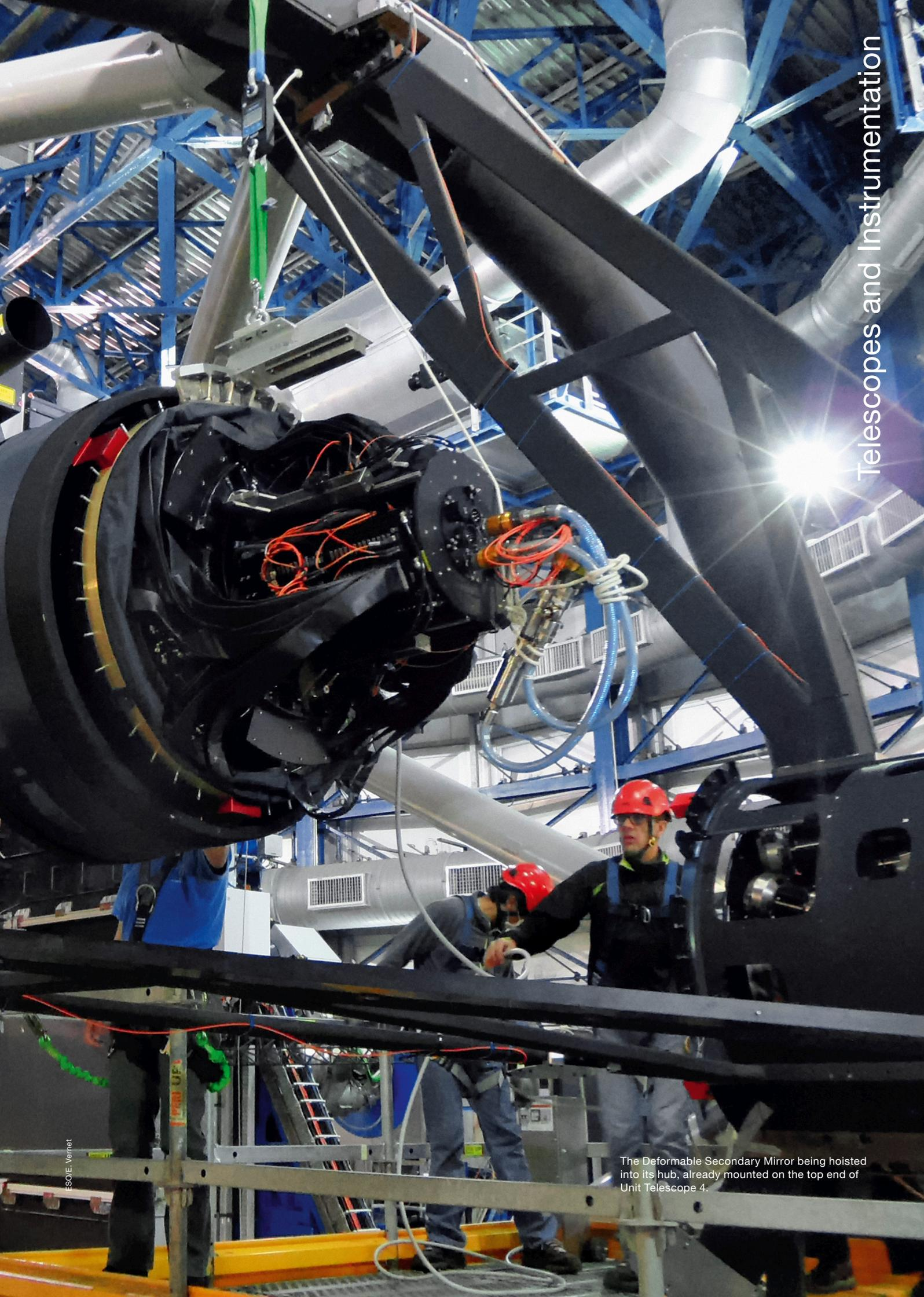
The Deformable Secondary Mirror being hoisted into its hub, already mounted on the top end of Unit Telescope 4.
