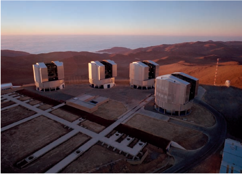
Figure 2: An aerial view of the Paranal platform as of December 1999, still in construction, with the four 8 m UTs and several foundations of the 30 stations for the 1.8 m ATs.
