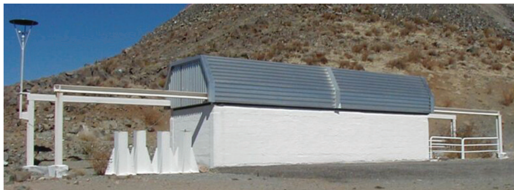
Figure 1: The GMS building, alias the "Sarcophago", located down the hill of the 3.6m telescope, in front of the new La Silla control room. It will host the TAROT-S experiment (photography M. Lopez / CNRS).
