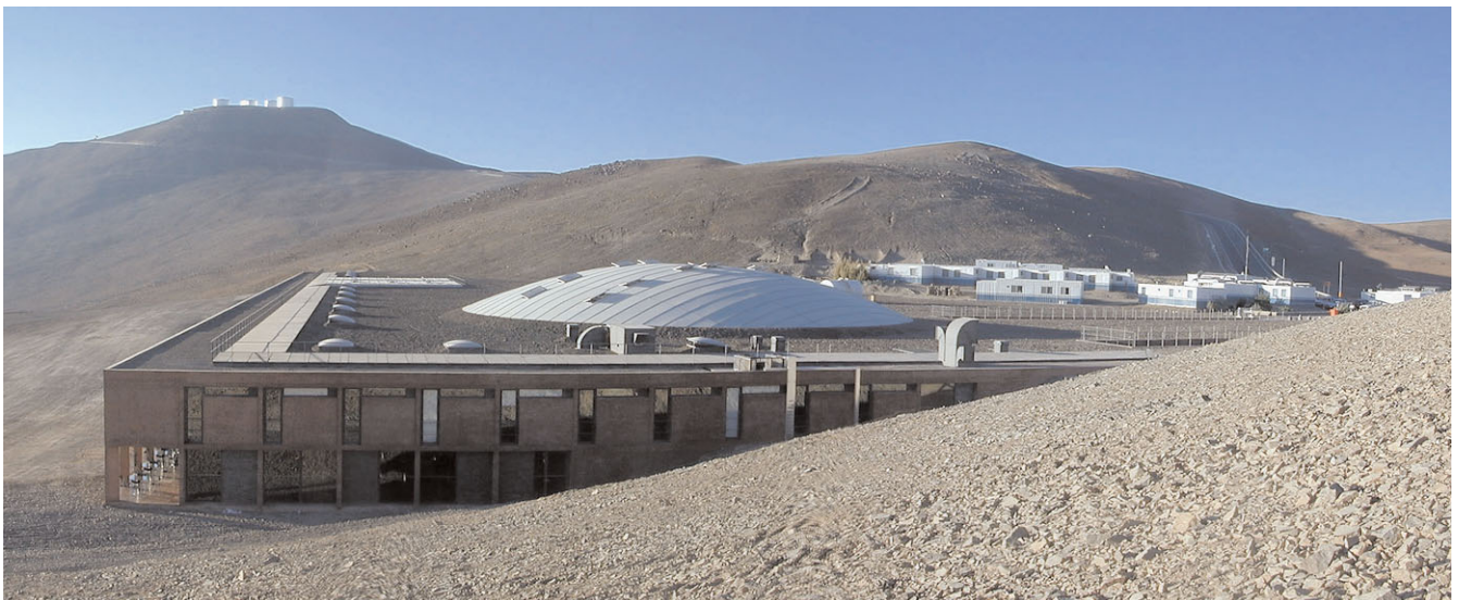
This photo shows the Residencia, looking towards west. The linear construction used to fill the natural depression of the ground in this area is evident. The 35-m central dome protrudes from the “filled-in” valley. Photo: Massimo Tarenghi.
