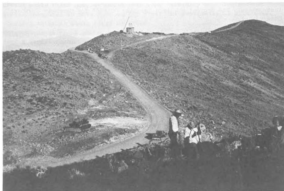
Fig. 2 Erection of building for 40-inch telescope.
