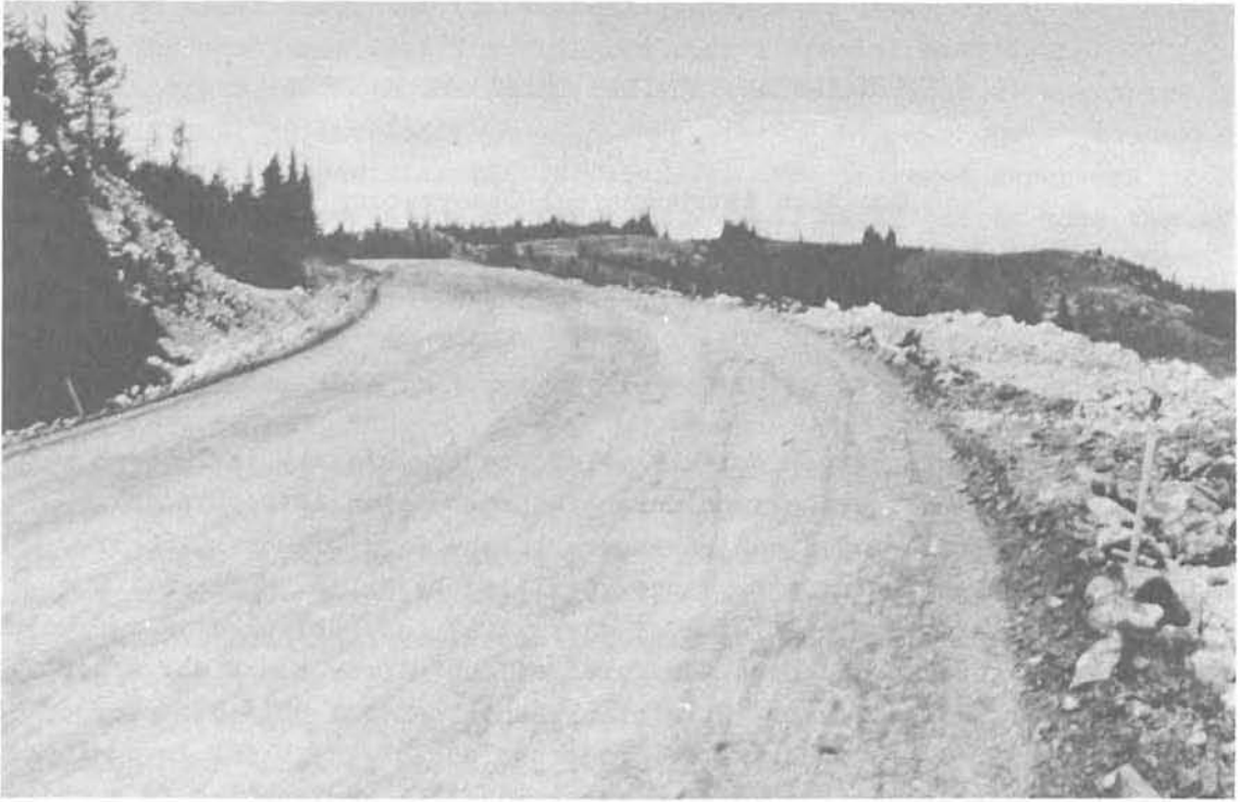
Fig. 1 Mount Kobau access road.
