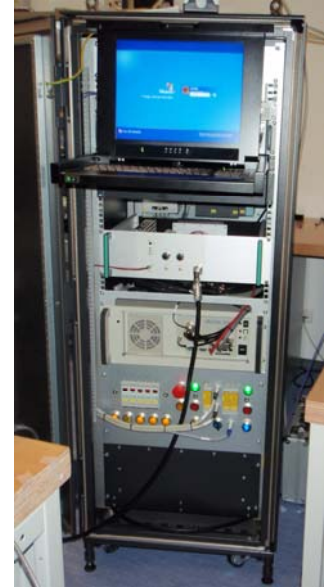
Figure 10: Electronics cabinet with the EOM RF driver, the integrated PC computer, the interlock panel, the EOM and AOM RF generators
