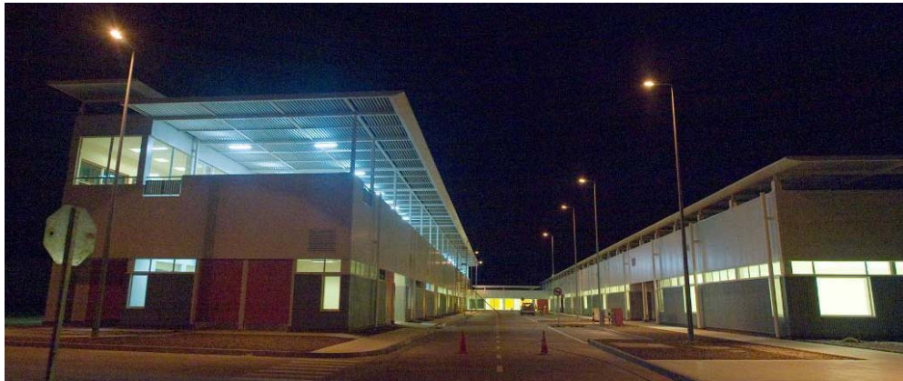
Fig. 4. Buildings at the Operations Support Facility (altitude 3000m).
