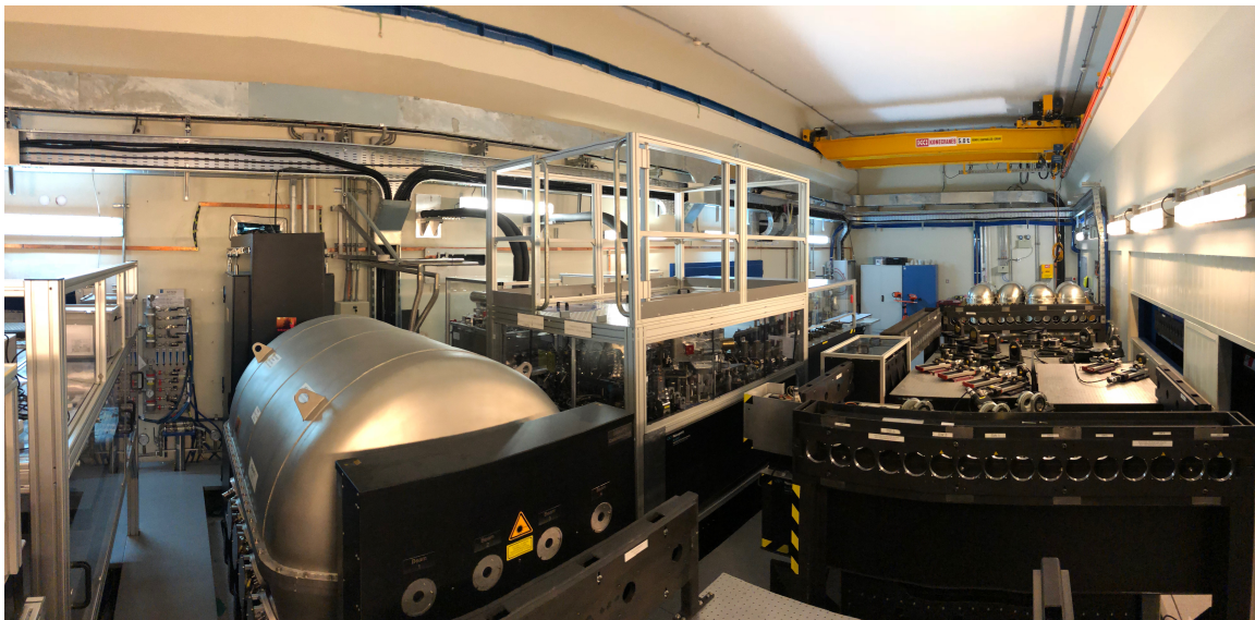
Figure 11: VLT lab: Top: drawing showing the main sub-systems. Bottom: Picture of the same elements taken next to the GRAVITY feeding optics.
