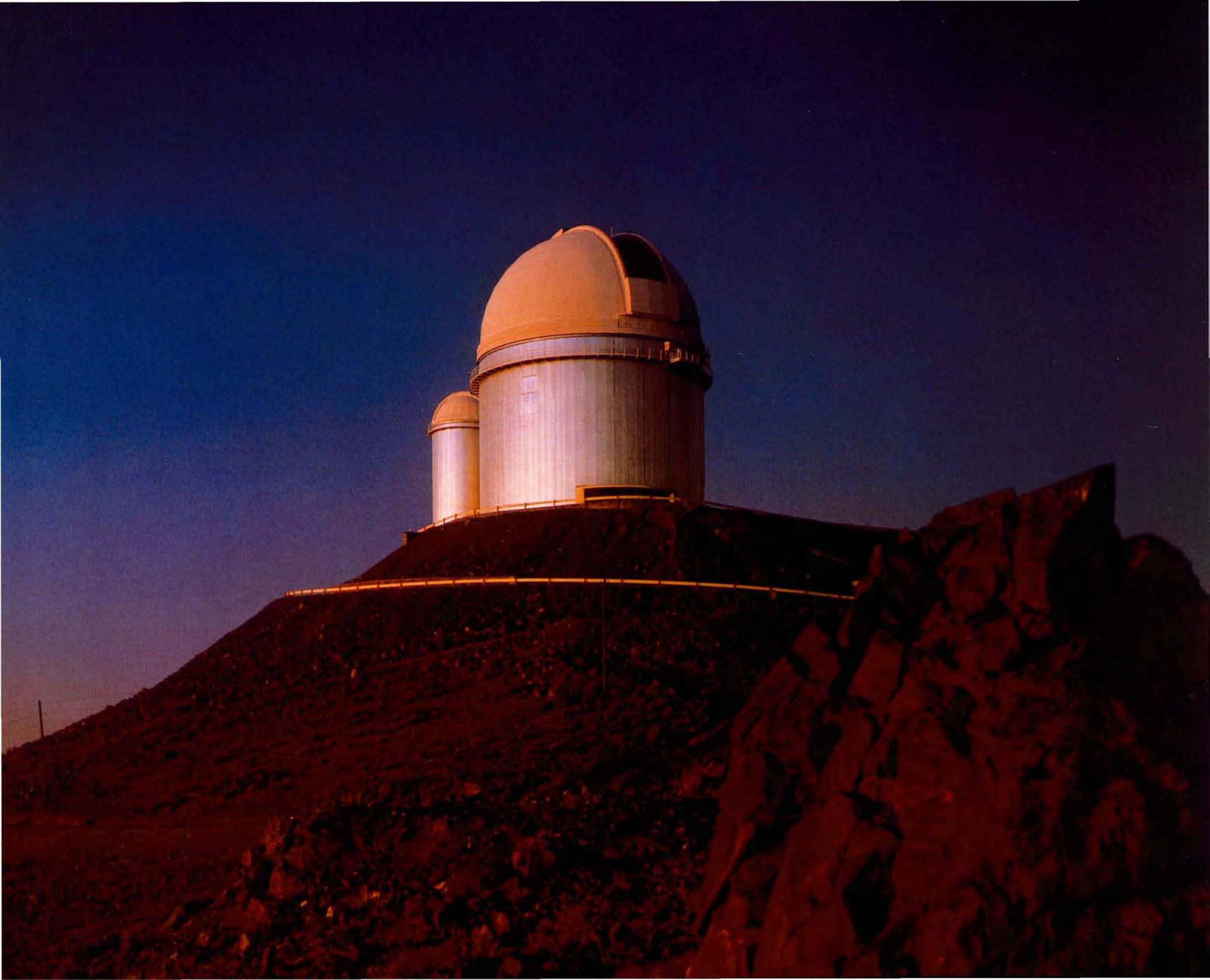
**214–215** The impressive dome of the 3.6-m telescope, here seen shortly after sunset, houses one of the largest reflectors in the world. The primary mirror weighs 11 tons and is made of fused silica. It was cast by the Corning Glass Works in the U.S.A. and the painstaking figuring was done by *R.E.O.S.C.* in France. The telescope is of the type known as a Ritchey-Chrétien and rests in a fork mount. The dome has a diameter of 30 m and a height of 45 m.
