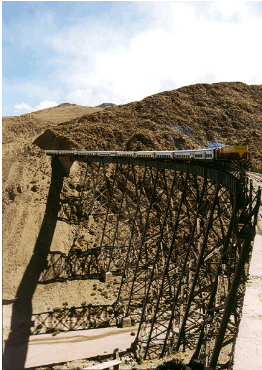
Train crossing “La Polvorilla” railway bridge near SAC.
